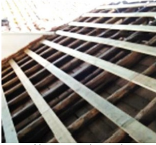
Nave central com ripas
